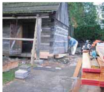
Repairing log cabin foundations.
